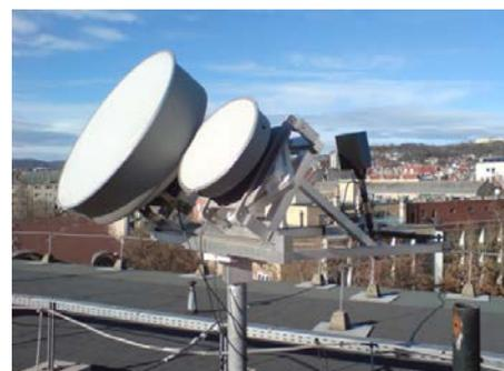
Figure 1. High performance antennas with tracking system
